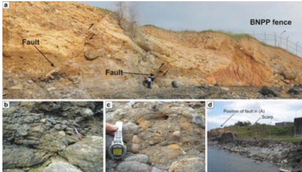
Figure 7. Evidence of faulting at the BNPP site. (a) 25 m-high outcrop of faulted lahar deposits. (b and c) Close-up photographs of rock masses sheared and deformed by faulting. (d) Scarp extending in the NNE direction from the faulted outcrop into the BNPP fenced perimeter. The BNPP facility is at the far right. From Lagmay et al., 2012 3 .
